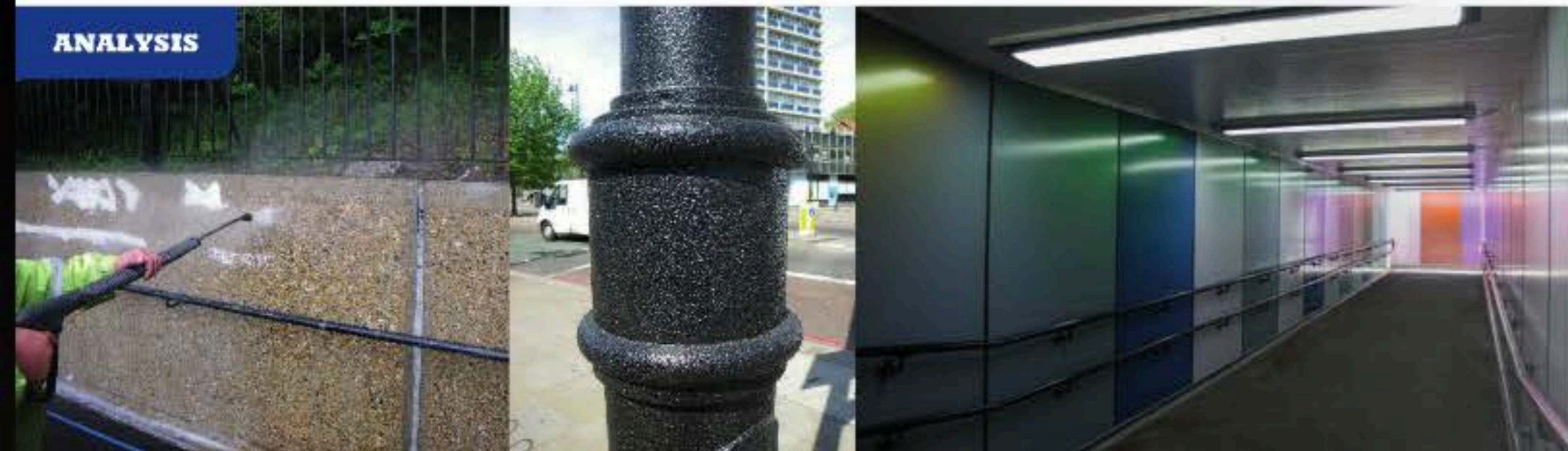
Left to right: Graffiti removal is estimated to be costing the UK over £1 billion a year; Anti-fly posting coatings are being tested; Rockpanel's Chameleon boards contain a crystal layer that allows them to dramatically change colour depending on the angle of view
