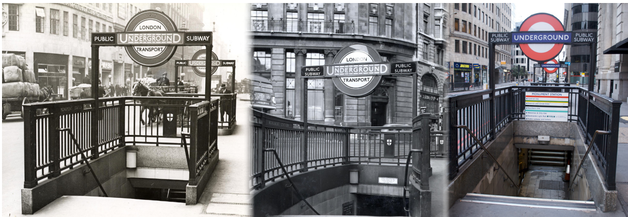
Monument Subway through the ages: 1936; 1955, and today
