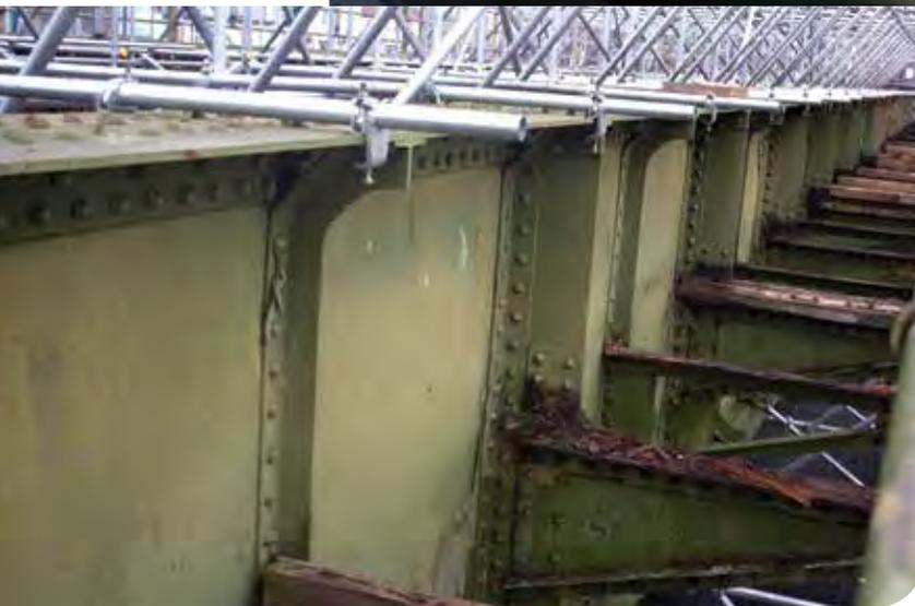
Above: Over 400 individual steel repairs were completed by a team of up to six welders
